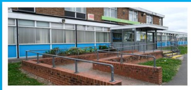
Horfield Jobcentre , 1, 15 Monks Park Ave, Horfield, Bristol, BS7 0UD: 2nd & 16th August
